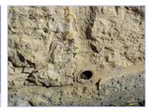
Stone retaining walls range from one to two feet in height and are used at the monument areas. Walls range are in overall fair condition with areas of grout loss and minor damage and movement noted. Funding is to repair and repoint walls as needed with no anticipation of replacing the entire wall.
