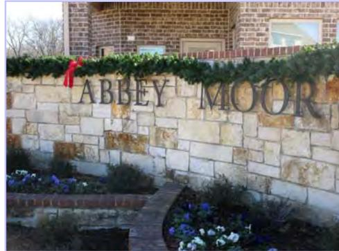
The entry monuments and corner neighborhood monument are constructed of stone with cut metal lettering. Funding anticipates periodic repair to stone work. Name plates will need occasional cleaning, paint, repair and replacement as well. Masonry should be inspected regularly and grouted as necessary to prevent moisture penetration which will accelerate deterioration.
