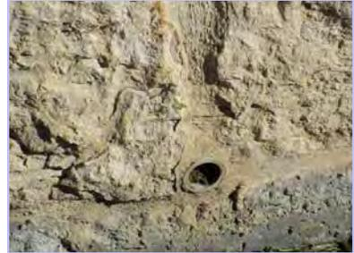
Stone retaining walls range from one to two feet in height and are used at the monument areas. Walls range are in overall fair condition with areas of grout loss and minor damage and movement noted. Funding is to repair and repoint walls as needed with no anticipation of replacing the entire wall. Drainage tubes were clogged in several areas and should be cleaned to maintain required water flow.
