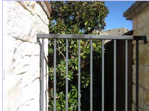
Metal fence is located at the corner neighborhood monument. Metal is in good condition with limited signs of decay or damage. Fence has a powder coated finish that once damaged will require restoring and protecting surface from moisture. Due to prohibitive costs of removing fence to re-powder coat, funding is based on maintaining fence by treating rust and painting. Recommend regular inspections to identify and treat damaged areas in order to avoid additional future costs to repair.
